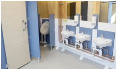
New fully accessible WC facilities
